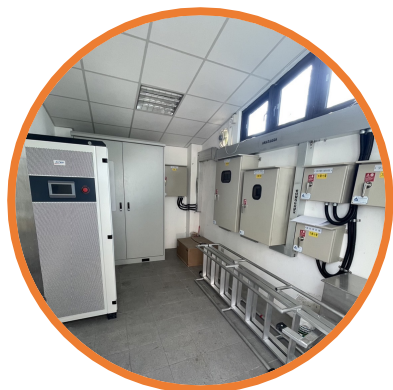
50KW/146KWh 鋰鐵電芯 (LFP)
