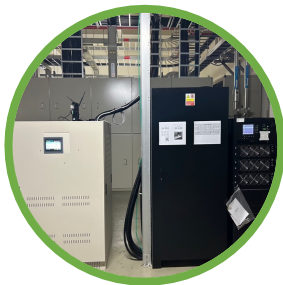
90KW/22KWh 鋰鐵電芯 (LFP)
