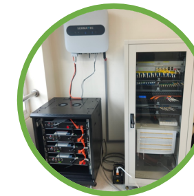
5KW/10KWh 鋰鐵電芯 (LFP)
