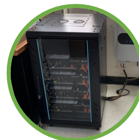
5KW/10KWh 鋰鐵電芯 (LFP)
