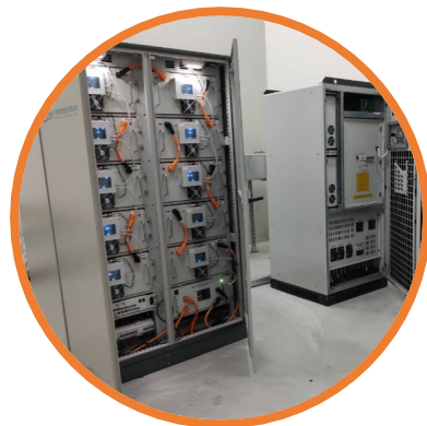
50KW/120KWh 鋰鐵電芯 (LFP)
