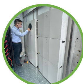
8KW/25KWh 鋰鐵電芯 (LFP)
